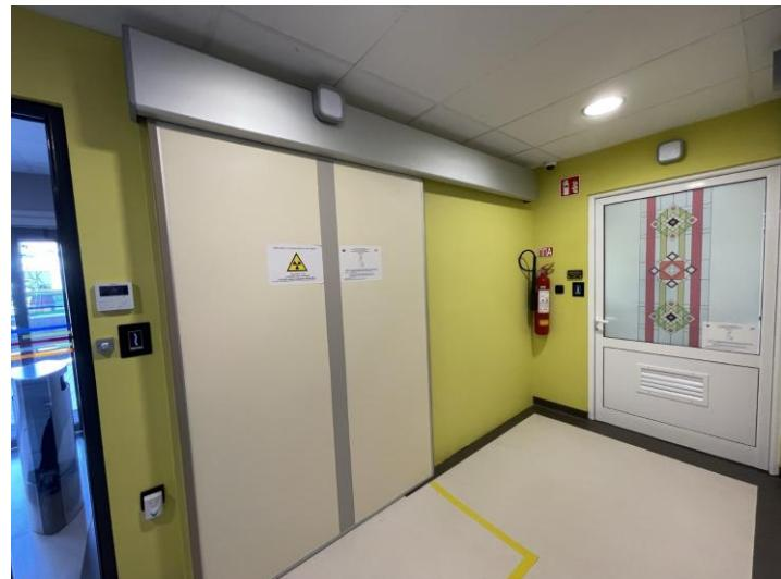
Atmas offers various options for hinged and sliding protective doors and gates for civil defence shelters, bunkers, safe rooms, industrial protected spaces and ammunition storage facilities and more.
