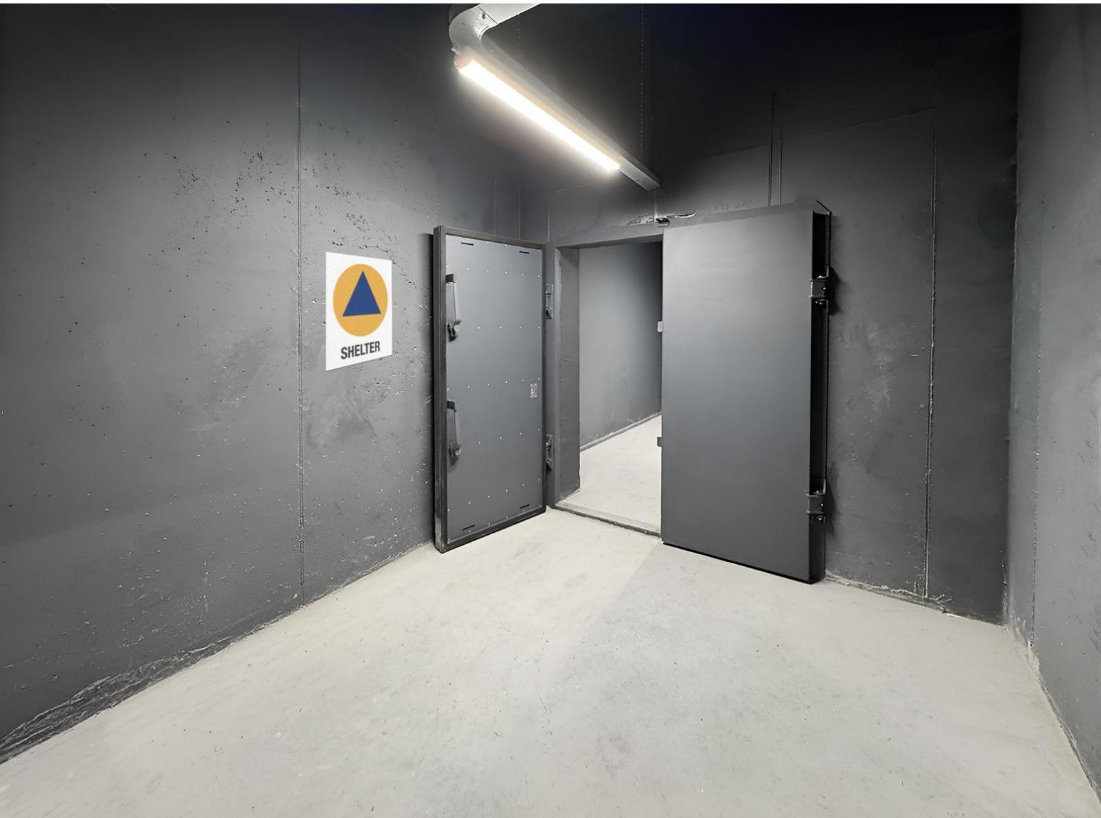
Atmas DU-III are part of a series of heavy-duty blast rated, and gastight doors designed for installation in civil defence shelters and protected facilities. The doors when installed in the shelter were designed to protect the internal space from blast wave pressure (in both positive and negative phase) and create gas tight shelter perimeter helping preventing harmful gases from entering inside.
